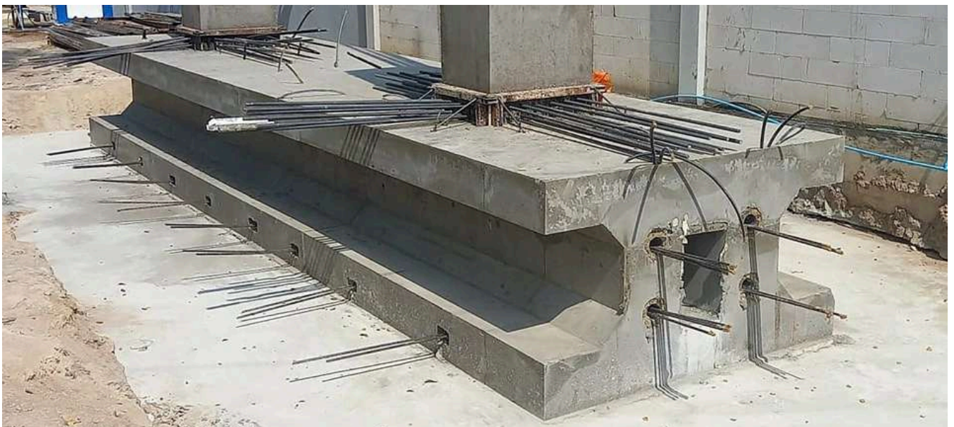
Post-tensioned concrete footing with visible tendons after casting, before stressing and finishing. Part of the integrated long-span structural system.
